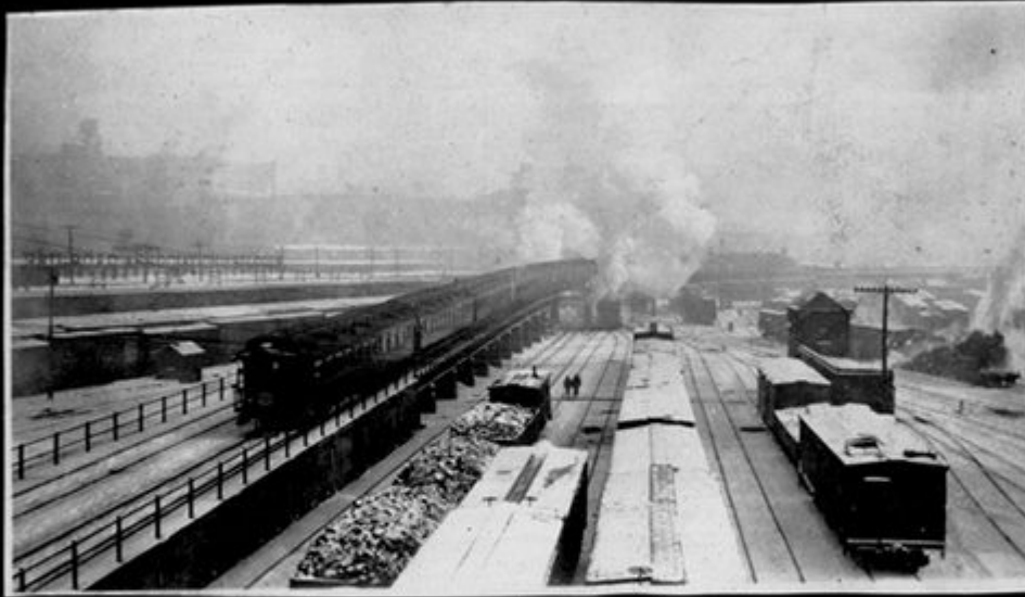
ST. LOUIS - JAN. 1915 Alton Ltd. ascending west approach to Merchant's Bridge elevated.
