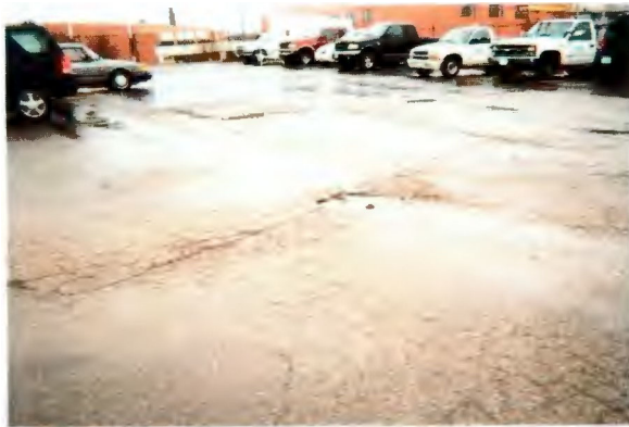
Alligator cracking and pothole in parking lot.
