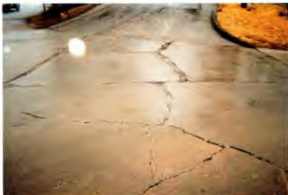
Cracked pavement on Stardust Drive.
