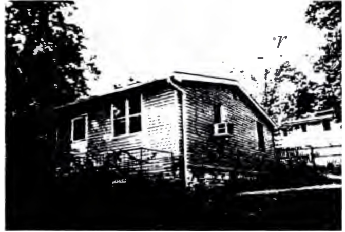
Deteriorated residential use with mildewed siding and boarded basement windows.
