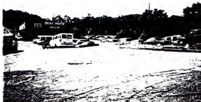
Deteriorated asphalt apron containing cracks and pot-holes. Note: parking lot excessively covered with vehicles and is unscreened.
