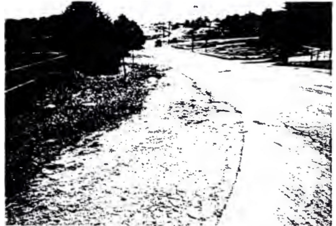
Big Bill road: crumbling asphalt, inadequate shoulder.
