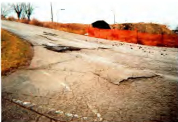
Deteriorated asphalt exhibiting severe erosion, potholes, and cracking at rear of 7-11 building.
