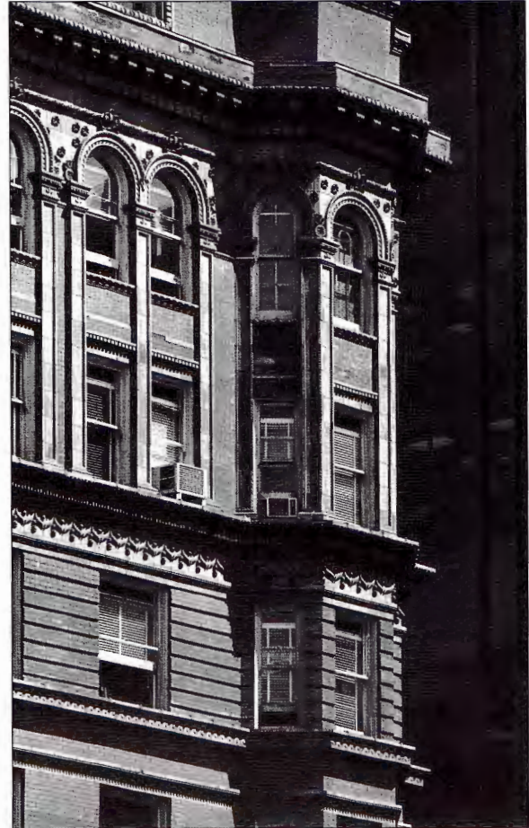
Detail: Chemical Building. Photo by Robert C. Pettus courtesy Landmarks Association.
