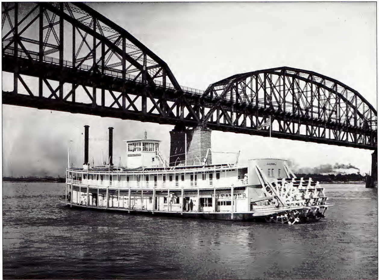
Merchants' Bridge with sternwheeler in foreground and steam locomotive in the background. Photo courtesy Landmarks Association.
