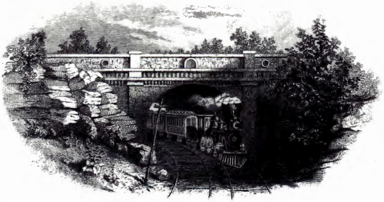
Entrance at Eighth and Spruce Streets to Eads Bridge tunnel from 1874 stock certificate courtesy Landmarks Association.
