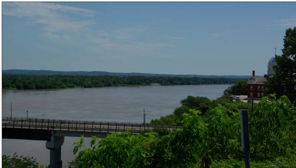
Senator Kit Bond Bridge on the Missouri River: Hermann, Missouri. Photo by Todd Brown.
