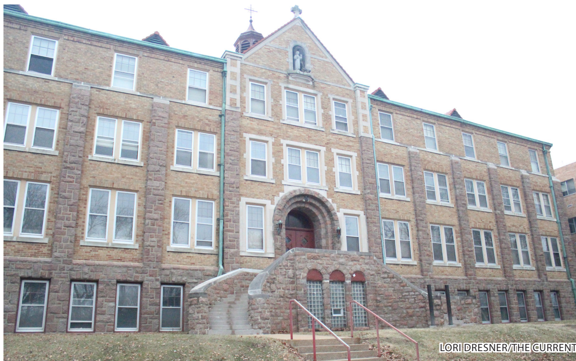
Normandie Hall's demolition is scheduled for 2015, due to a lack of maintenance funds
