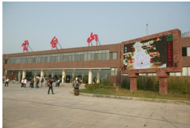
Figure 5.13 LED Information Distribution System
